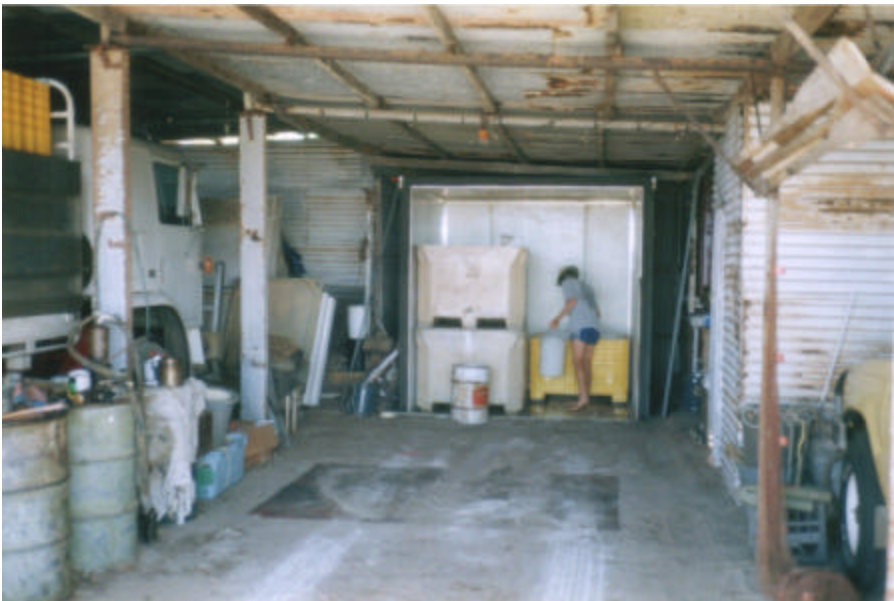
Cool room in shed, with room for 4x 0.5t bins with ice. Ron Heberle.
