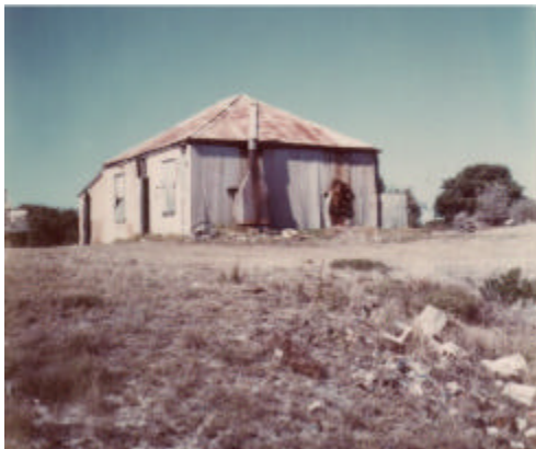
House at House Beach.
