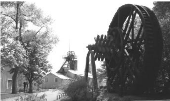
Kulturdenmal Oberharzer Wasserregal, Kaiser Wilhelm II Schachtes, Erzstrasse24, Clausthal. Water management facilities.
